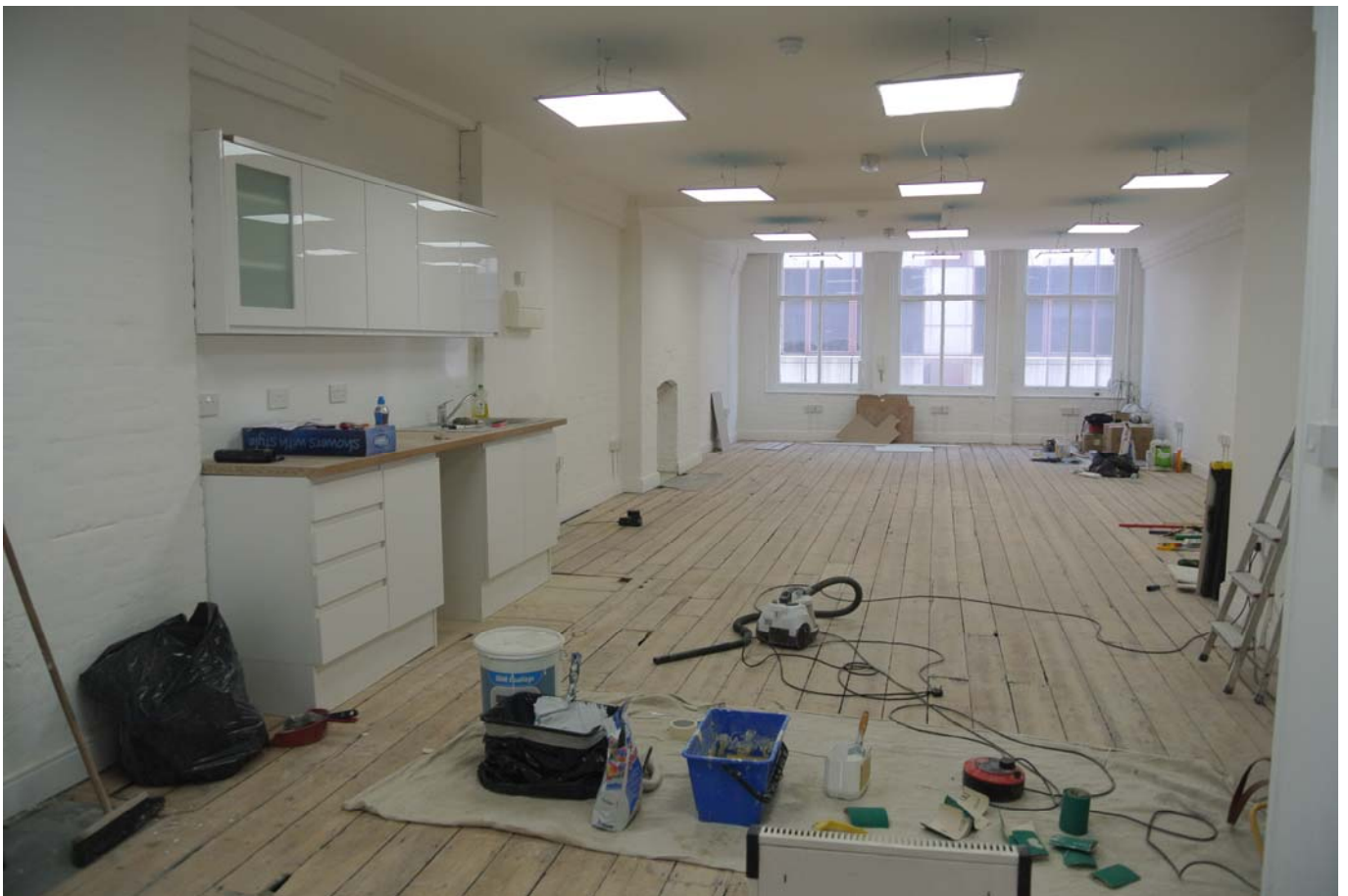
PHOTO TAKEN DURING REFURBISHMENT OF 2 ND FLOOR IN 2013
